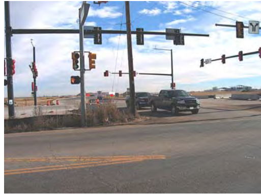
Recent construction along Quebec Parkway.
