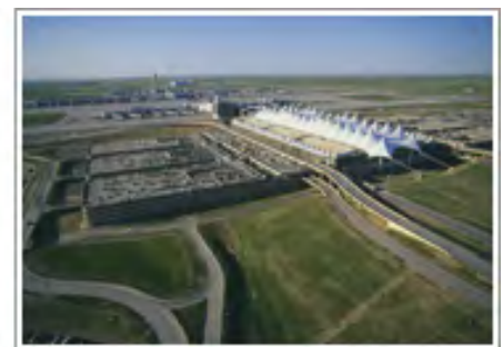
Denver International Airport.
